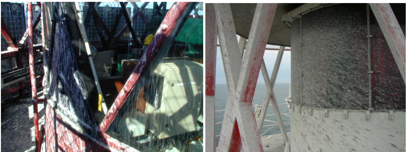
Figure 4 Examples of bird fouling accumulating on lighthouse glazing (Source: Trinity House and Danish Maritime Authority)
