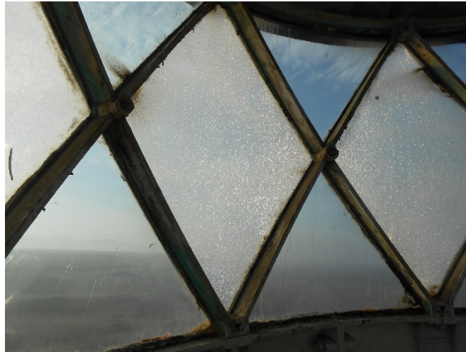
Figure 5 Example of different degrees of degradation of glazing panels made from plastic (diamond) and glass (triangular). Source: MSM
